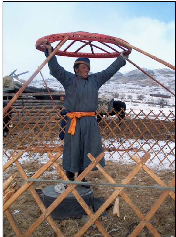
This ger has no support poles, so a herder holds the tono the entire time. In this case, there are no four ropes as guides.
