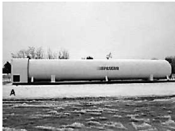
**Plate 7.** Liquid CO<sub>2</sub> vaporizer.
