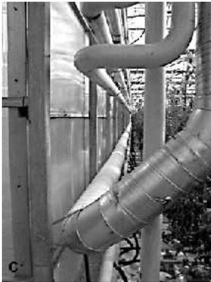
**Plates 3e.** Flue gas distribution in greenhouse.
