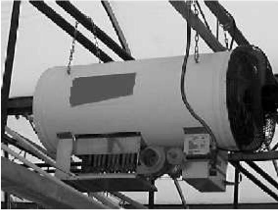
**Plate 2.** Hot water boiler with flue gas condenser.
