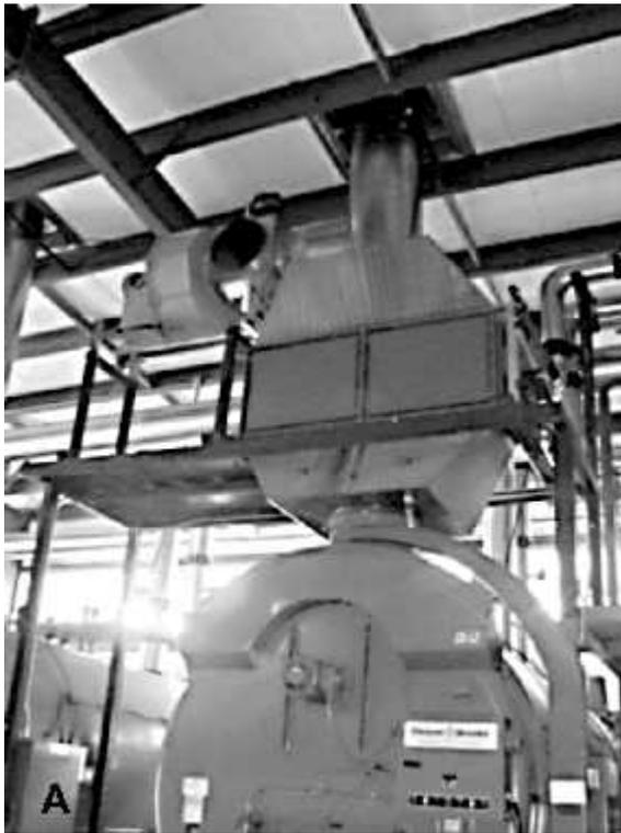
**Plates 3c.** Flue gas CO<sub>2</sub> distribution pipes.
