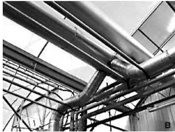
**Plates 3d.** Flue gas distribution in greenhouse.
