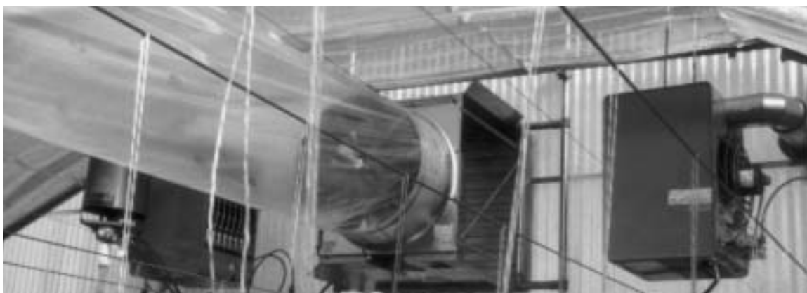
Traditional fan jet systems are commonly used to distribute heat produced by heaters and to recirculate inside air when the heating system is not in use.
