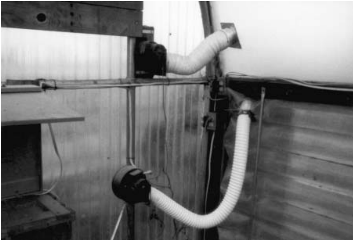
Small squirrel-cage blowers (¼ or ½ HP) can be used to inflate between the two layers of plastic covering the greenhouse. It is important to use outside air for this purpose so that condensation does not collect between the layers.
