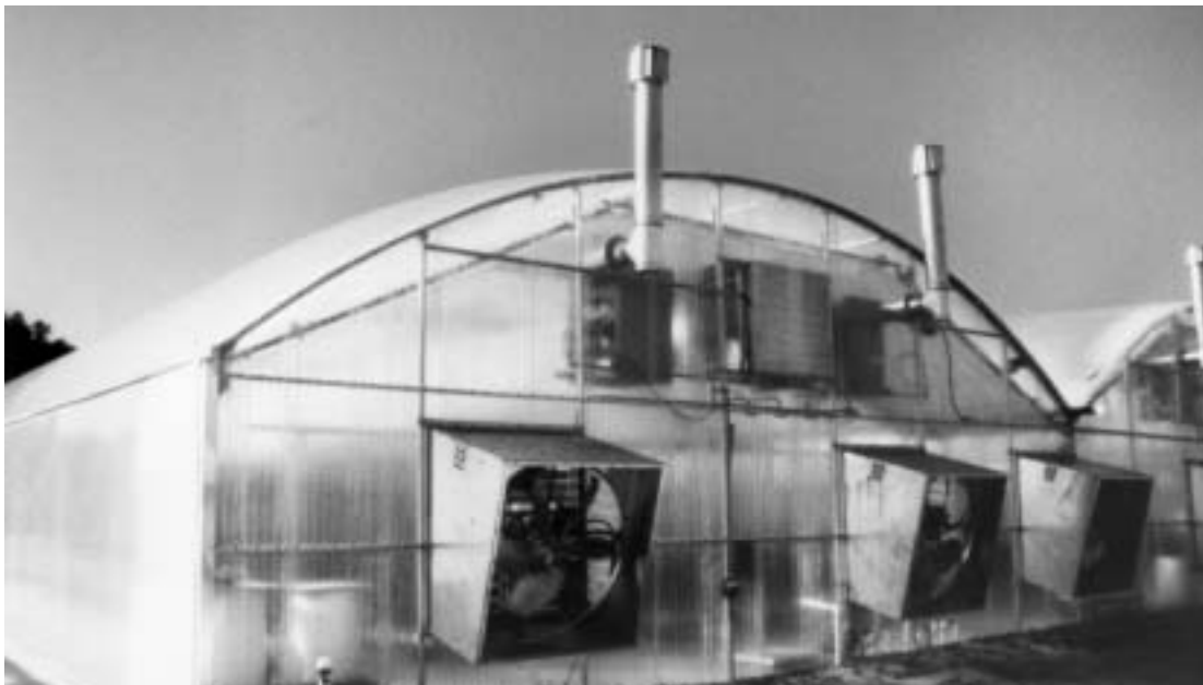
Proper sizing of the exhaust fans is important to ensure adequate temperature control during warm periods. Refer to the text for the simple calculations.
